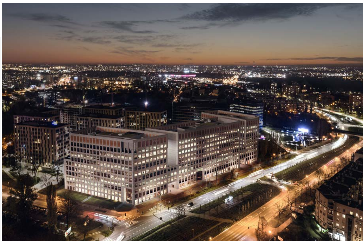
Brain Park office project under construction in Kraków.
